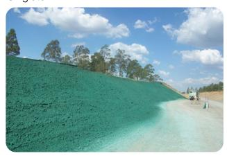
As can be seen, the compost blanket application has achieved 100% cover on the steep embankments to result in stabilisation of the surface. The bottom metre had to be reshaped, hence the lack of grass on the bottom of the batter.
